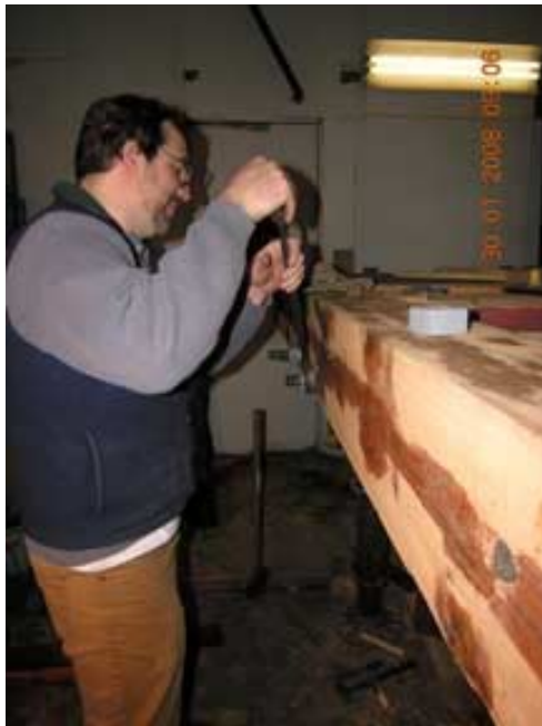
Randy tightening bolts on no. 2 end.
