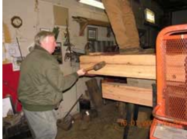
Donald Curry & Randy Leclair lining up the through-bolts to go through the end sill. Norman Down giving a little help to getting it in place.
